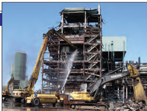
North American Dismantling
