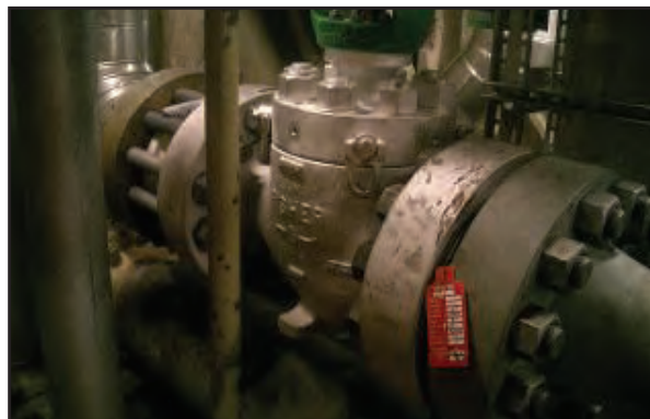
FIGURE 1. This picture shows an example of an anti-surge valve
